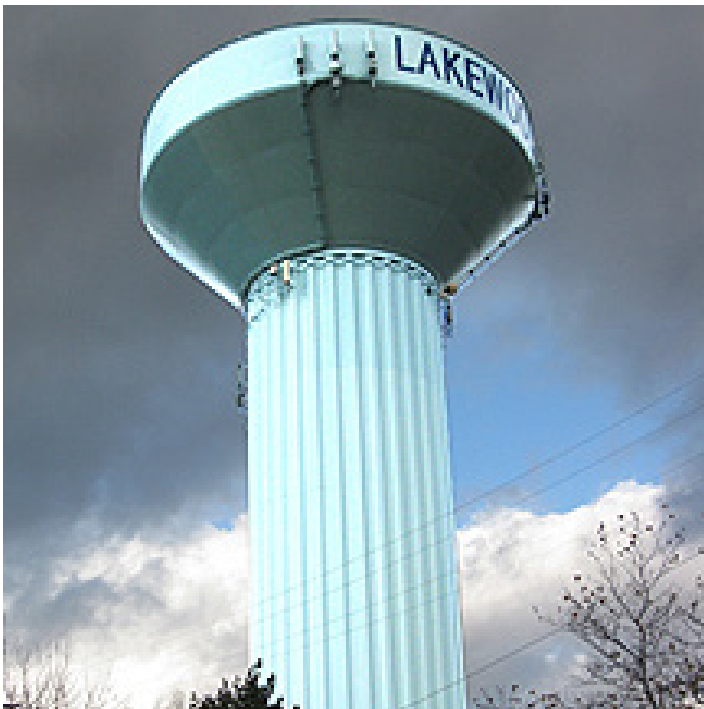
Lakewood water tower
