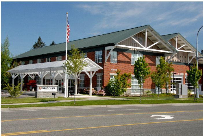
Station 20 Shortly After Construction (2004)
