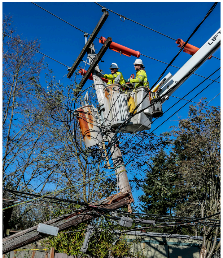
PSE crews repairing downed power lines in Lakewood
